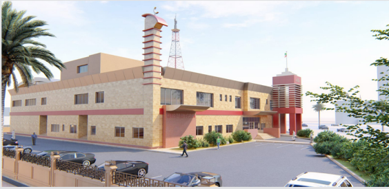
Fire Station - AL Jahra
